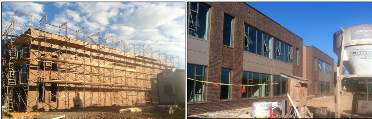
Figure 1: Installed Masonry Scope & Scaffolding (Property of Mascaro Construction)
